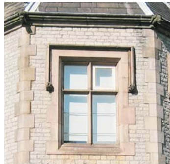
(j) Carved stone, including window/door surrounds, mullion, quoins and hood moulds.
