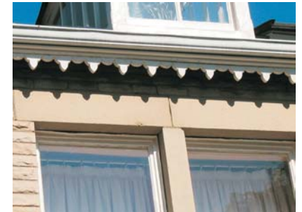
(l) Stone sills and lintels.
